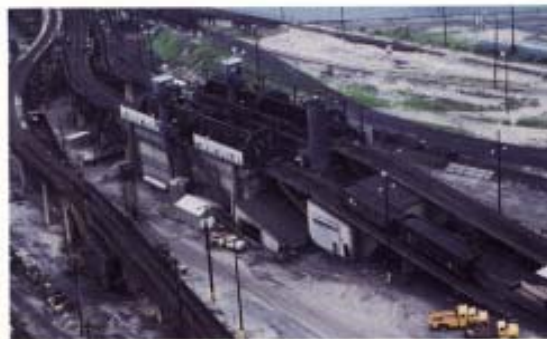
The tandem rotary dumpers receive the hopper cars and rotates them 165°, dumping the load into blending bins. To protect the environment, a mist of water covers the dumping coal to stop any dust.
