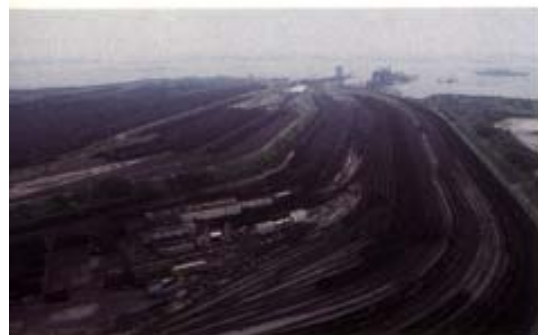
The massive switching yards hold some 4,000 coal cars, loaded and empty, in the 400 acre complex of Lamberts Point facility.
