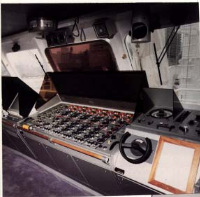
The bridge of WIND SONG , with the computer console that controls the furling and unfurling of the sails.
