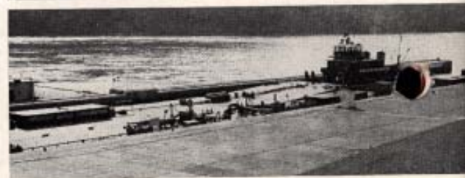
Left: Starboard bow view of our Betty on the Mississippi River below St. Louis. Note characteristic pushing knees and 12-foot radar scanner.
