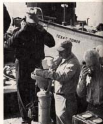
Control point aboard tower, at a critical moment it was about to be pinned to the seabed. Capt. Frank J. Hughes, Henry Camus and Harry G. Steers and Morrison-Knudson, and other key personnel were vital factors in a "must" here.
