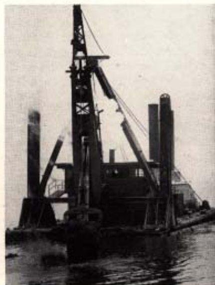
Schultz Dredging Corp.'s three-cubic-yard dipper dredge Kingston , at work
