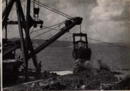
American Dredging Co.'s clamshell Camden
